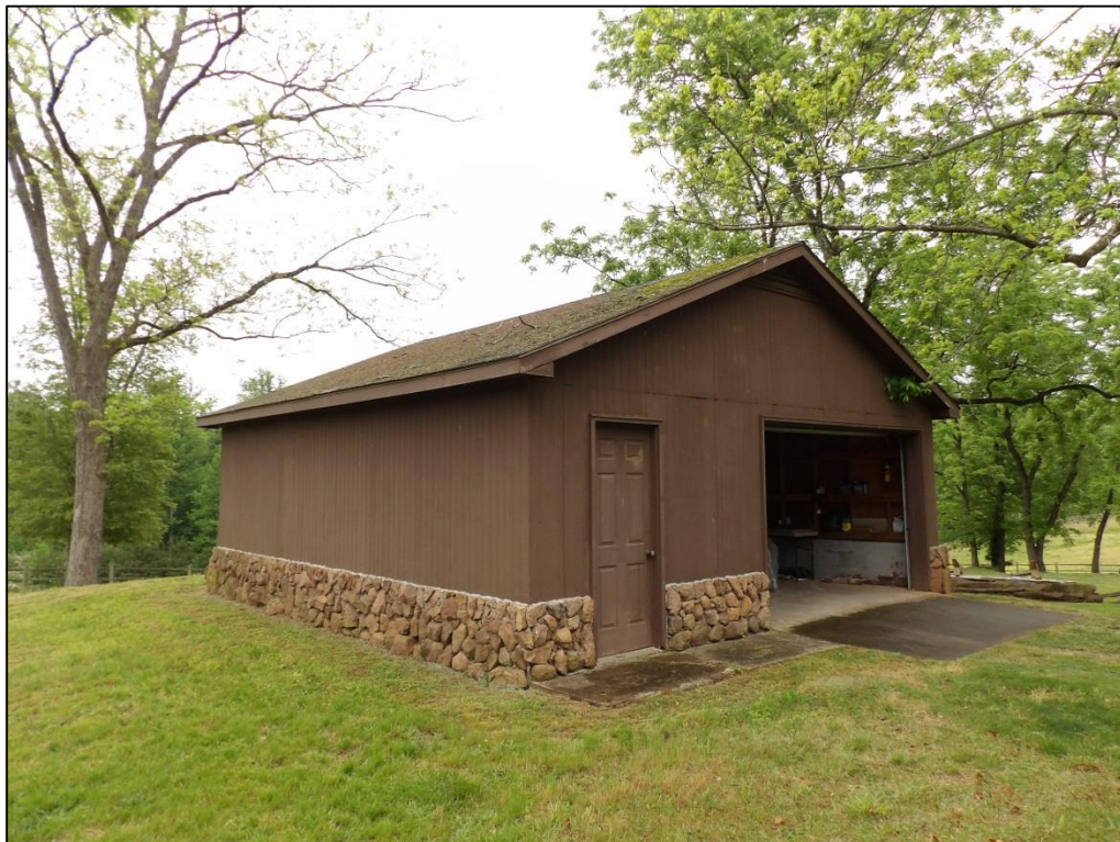
Photo 23: Garage, Looking Southeast.
