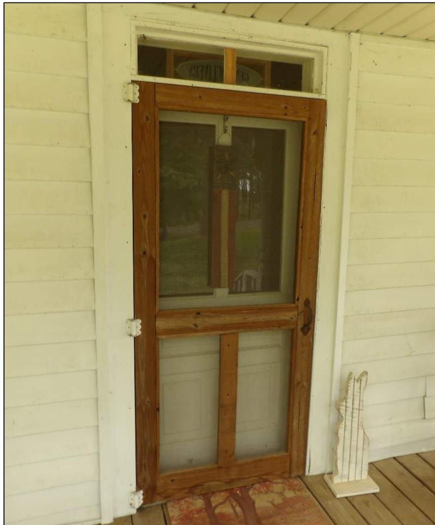
Photo 13: Entrance on the West Elevation of the 1902 Addition, Looking East.
