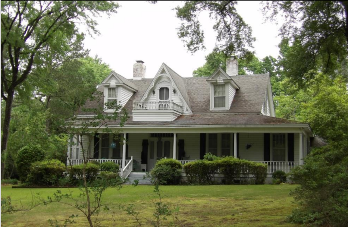
Photo 34: House at 108 Sanford Street, Carthage, Moore County, North Carolina, Looking Northeast.
