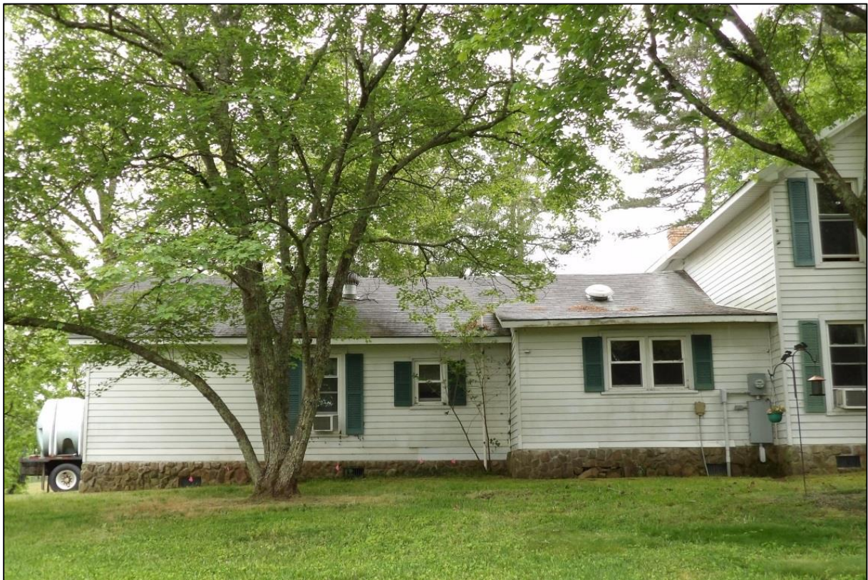
Photo 2: North Elevation of Original Log Section and One-Story Addition, Looking South.
