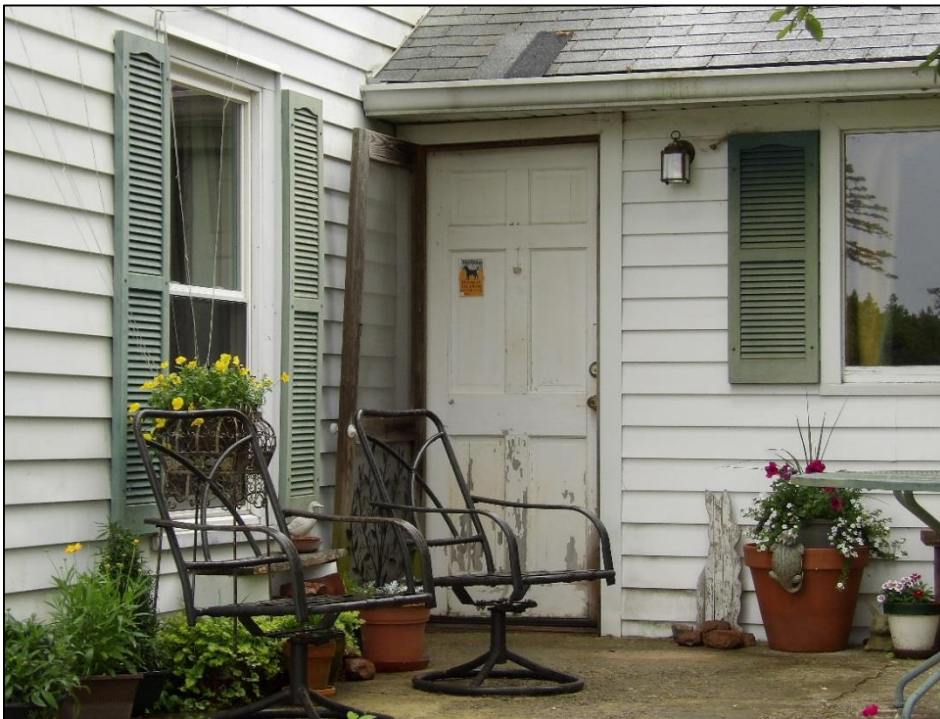
Photo 18: Entrance on the South Elevation of the One-Story Addition, Looking North.
