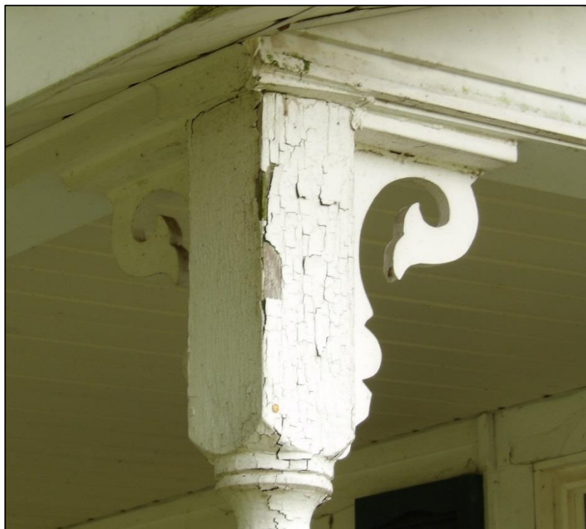
Photo 15: Detail of Scrollwork Brackets on Porch.
