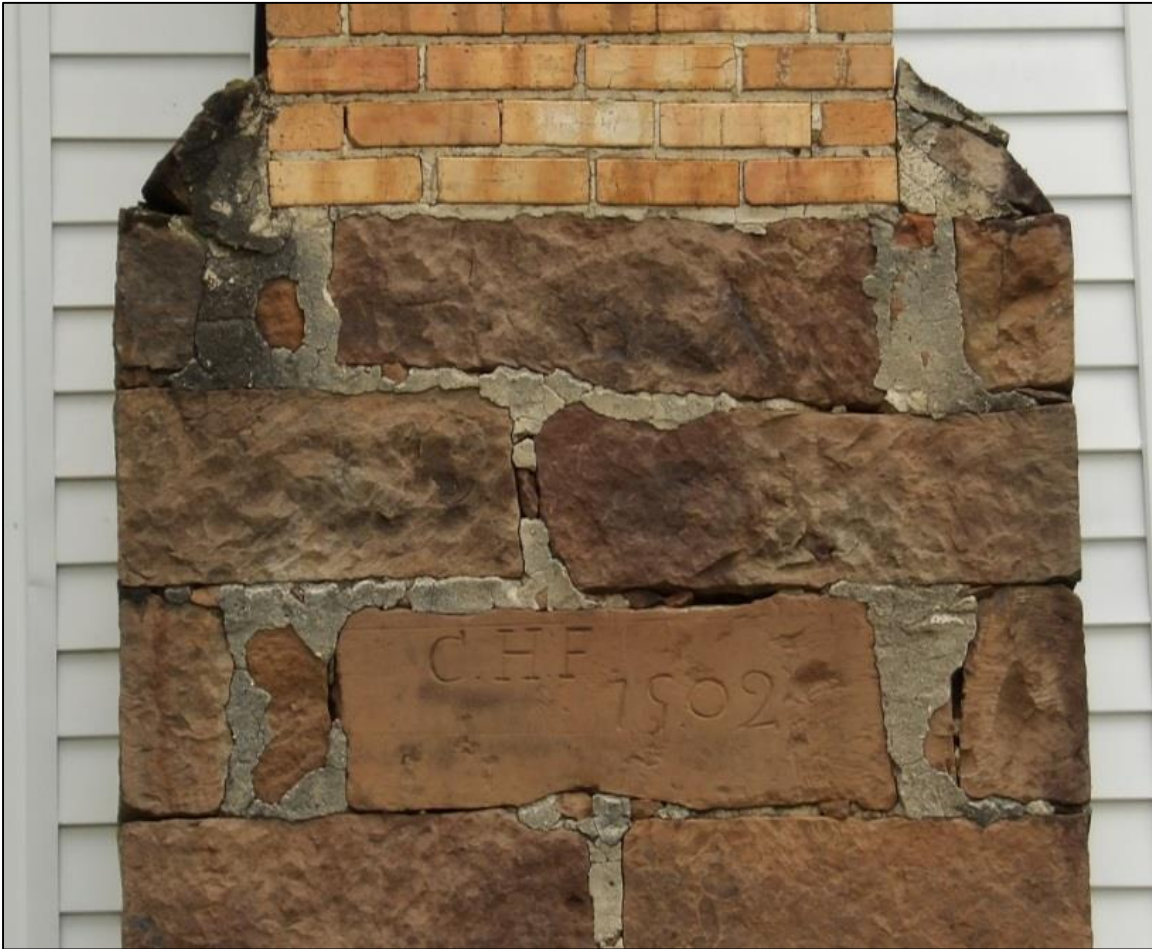
Photo 12: Detail of Composite Masonry Chimney on Two-Story Addition, Showing Date Stone.
