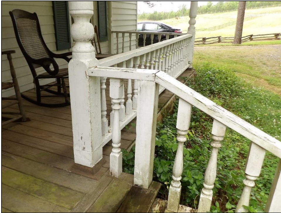
Photo 14: Detail of Porch, Showing Replacement Balusters and Handrail, Looking Southeast.
