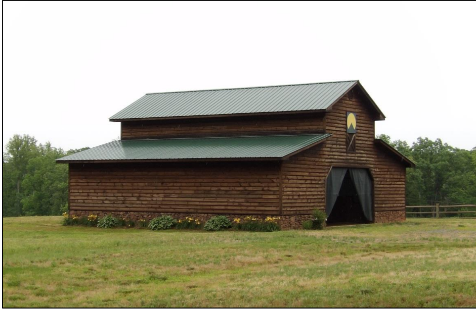
Photo 24: Horse Barn, Looking East.
