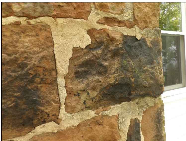
Photo 6: Detail of Chisel Marks on the Stone Chimney, Looking Northeast.
