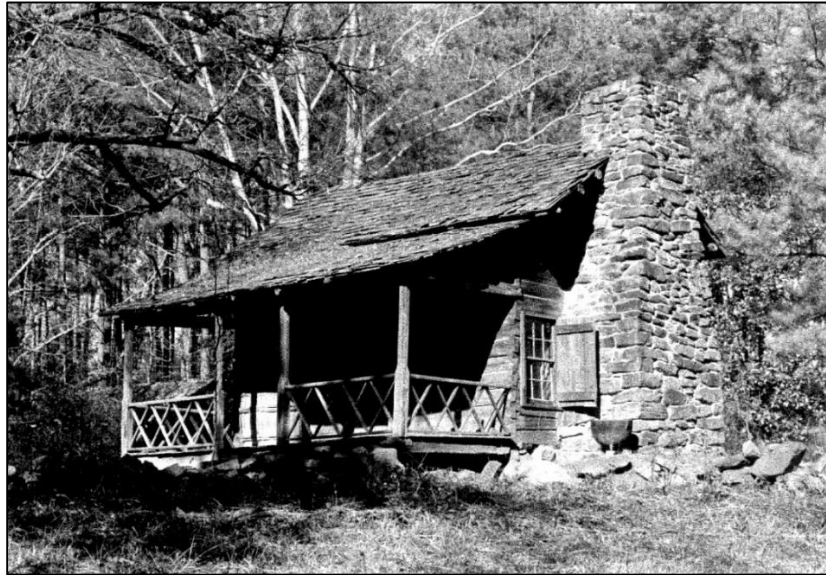
Photo 25: The McLendon Log House (MR0009) in Moore County, North Carolina. 64
