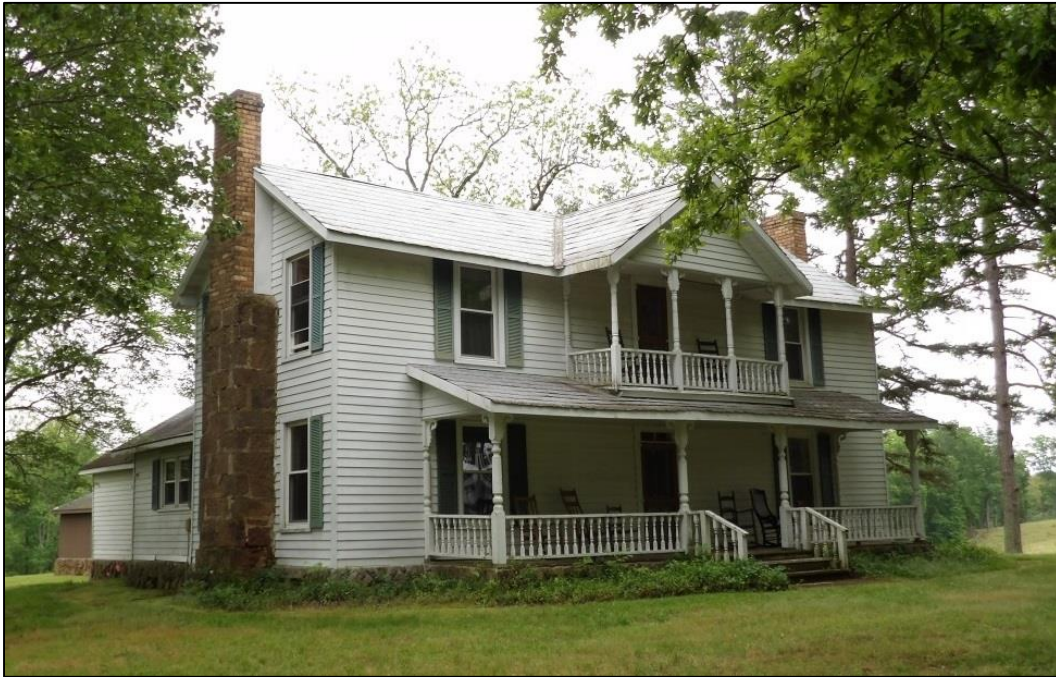
Photo 3: Northwest Oblique of 1902 Two-Story Addition, Looking Southeast.
