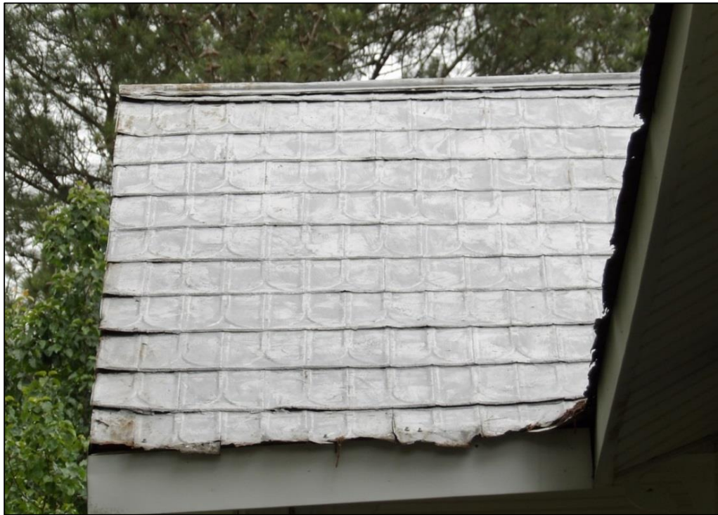
Photo 11: Detail of Pressed Metal Roof on Front-Facing Central Gable, Looking North.
