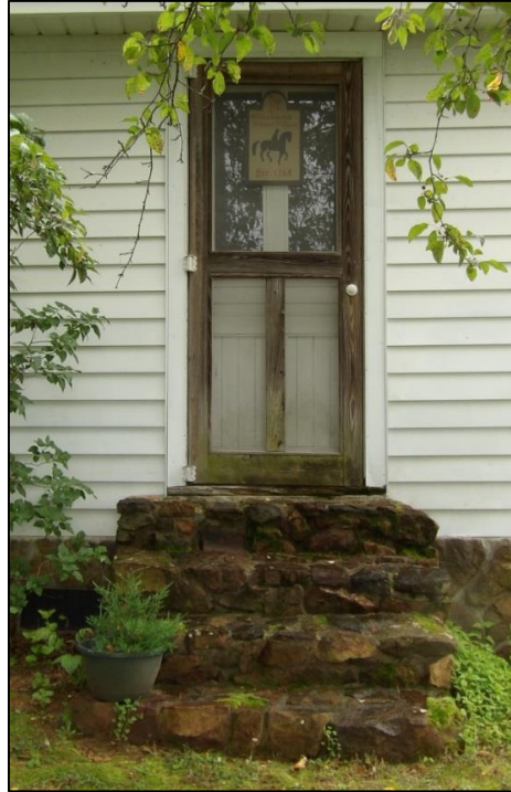
Photo 7: Entrance on South Elevation of Log Section, Looking North.
