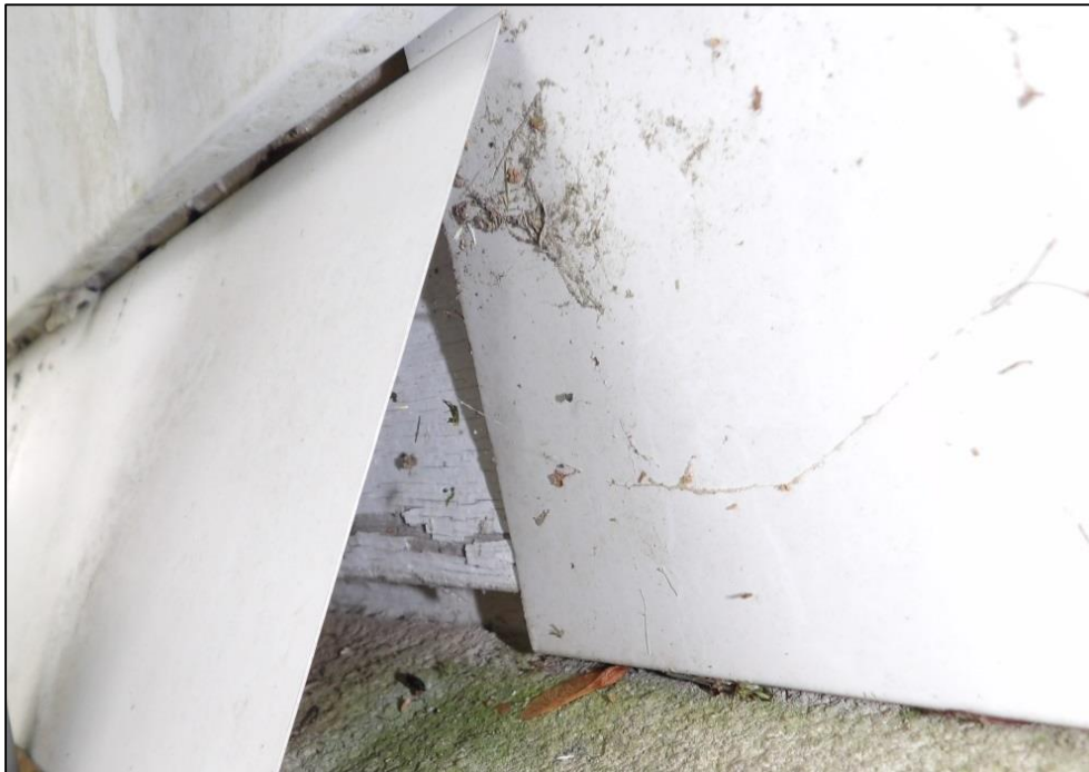
Photo 9: Wood Siding on the North Elevation Visible Under Loose Vinyl Siding.
