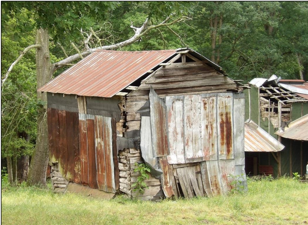
Photo 31: Log Outbuilding Associated with the Wadsworth Log House, Looking Southeast.
